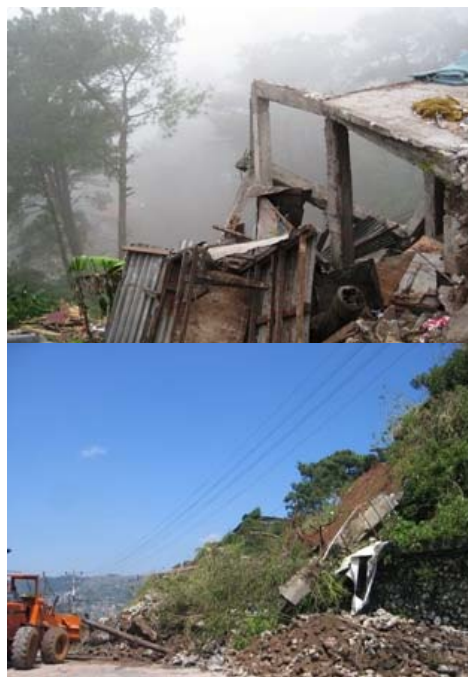
Wrecked houses in Bakakeng Central and Bokawkan Road, Baguio City
